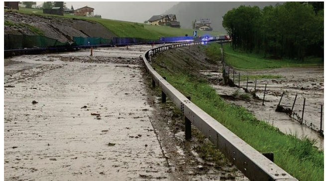
The highway A13 in Grisons, Switzerland is closed due to flooding and landslides (June 2019; photo: KEYSTONE)
