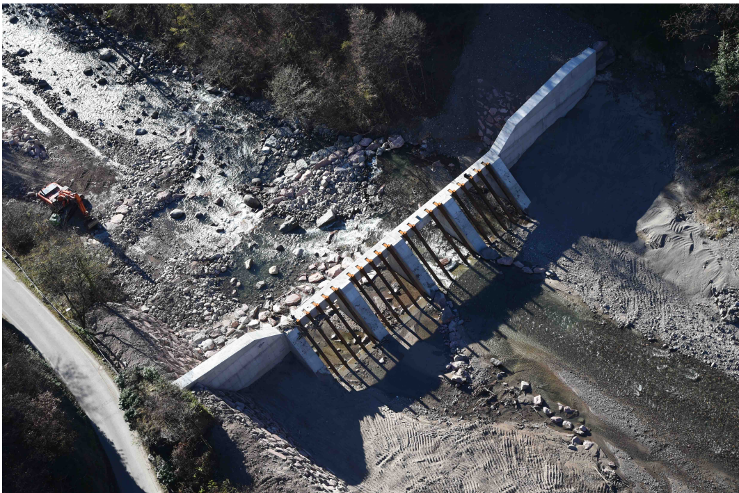
Figure 3.3: The new slit dam built in 2018 - the steel filter
