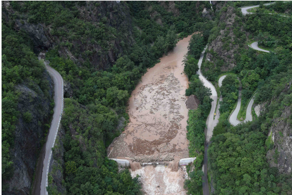
Figure 3.6: The new slit dam during the August 2021 event
