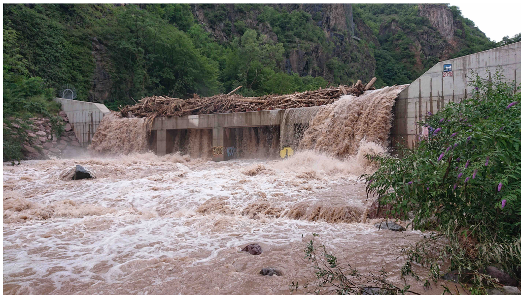
Figure 3.5: The new slit dam during the August 2021 event
