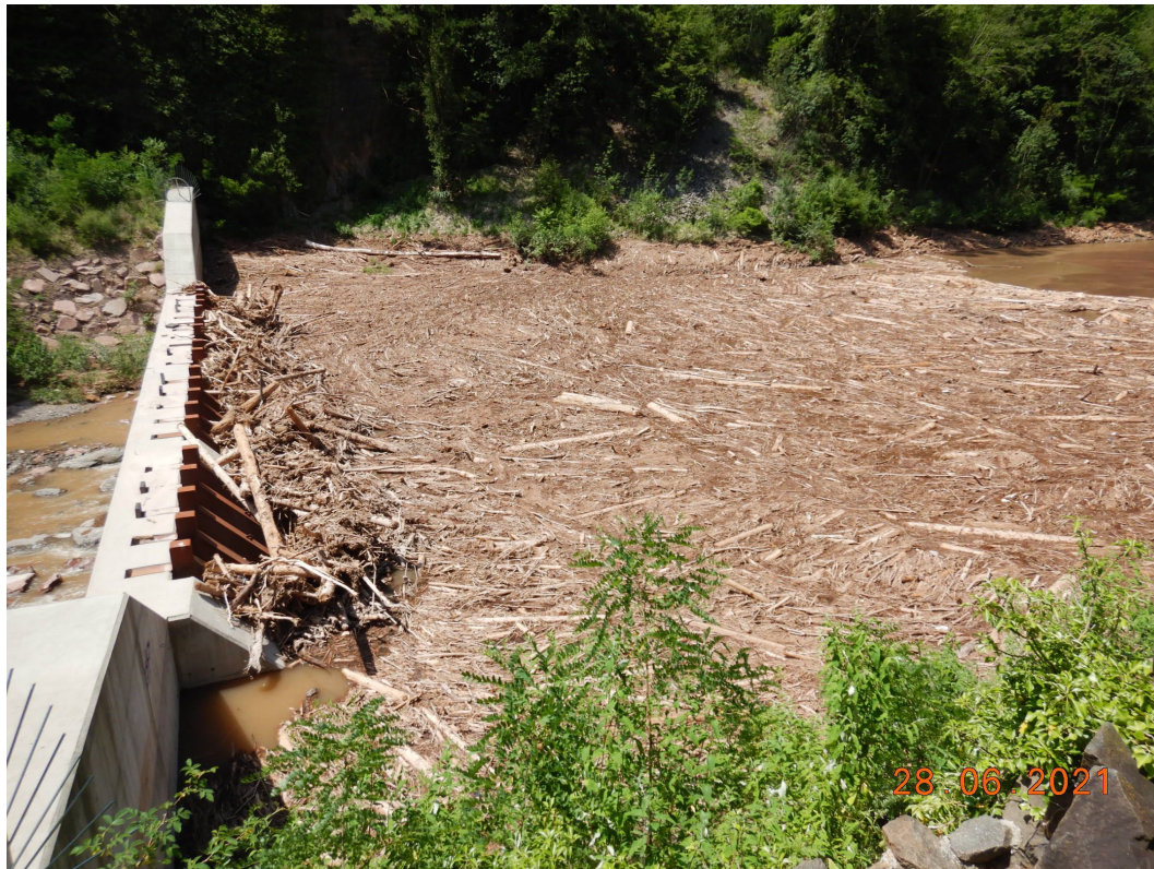
Figure 3.4: The new slit dam during the event of June 2021
