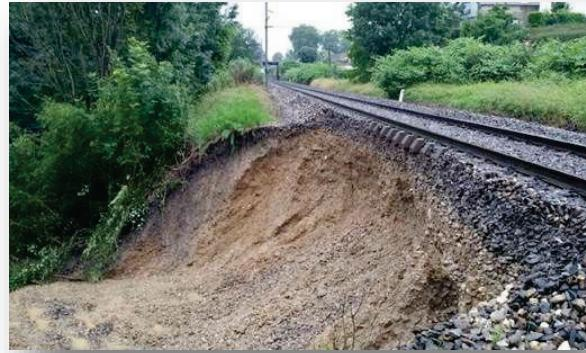
Railway between Chambéry and Lyon endangered by a shallow landslide (June 2018; photo: DR SNCF)
